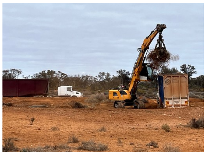
Three 3-ton loads were removed from the old dam site
