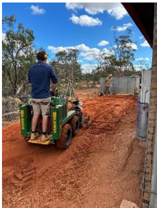
Preparing for the concrete
