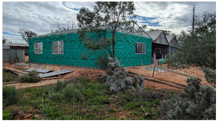
Walls and roofing form the shape of the new structure.
