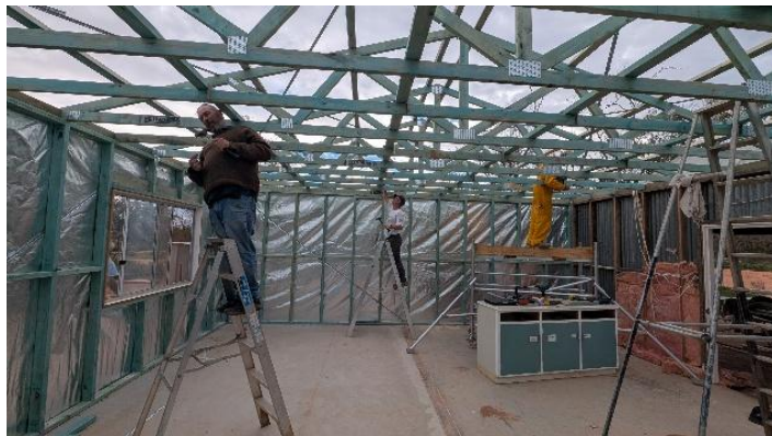
Enclosing the walls once roof trusses are in place
