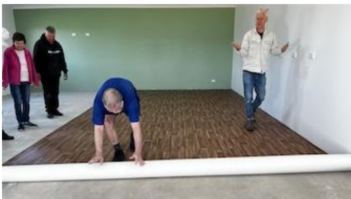
Placing the first roll of lino along a marked line
