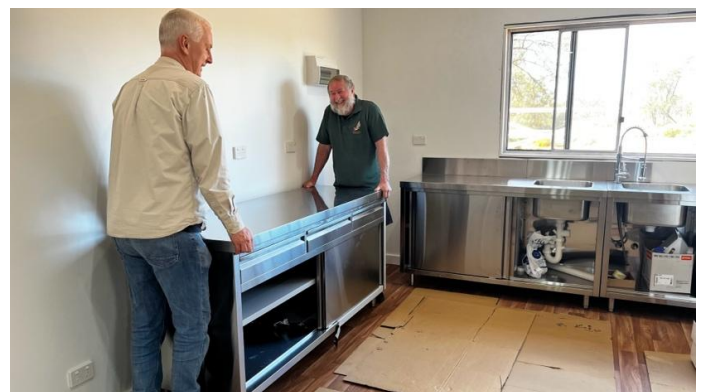
Bringing in the first kitchen fitting
