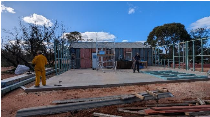
Initial stages of extension with one original wall remaining
